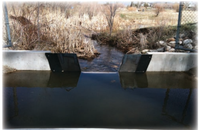
MARTIN SLOUGH WEIR
